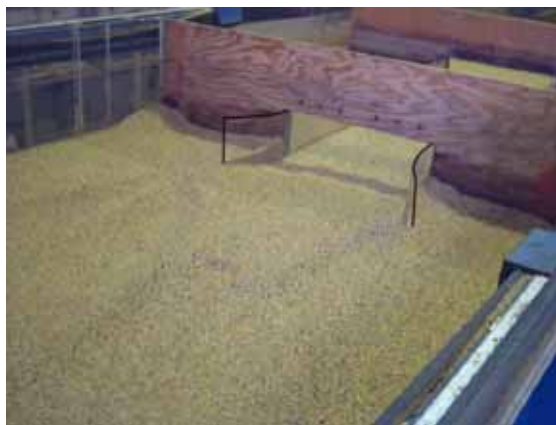
Figure 35. Photo. Short, streamlined bevel wingwalls after scour.
